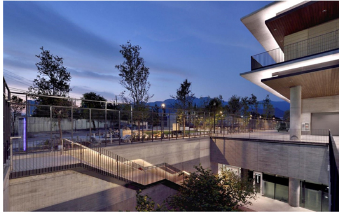
Estadio Banorte - Borregos, Monterrey, Mexico Built with Fortis and Promptis concrete, part of our Vertua family of sustainable products
