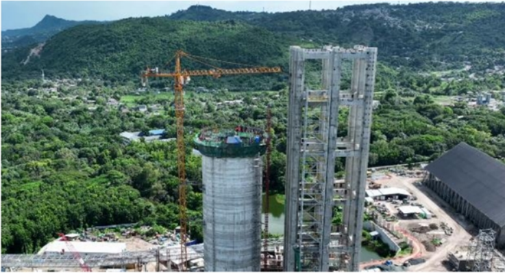
Preheater and silo under construction in Solid Plant New Line project.
